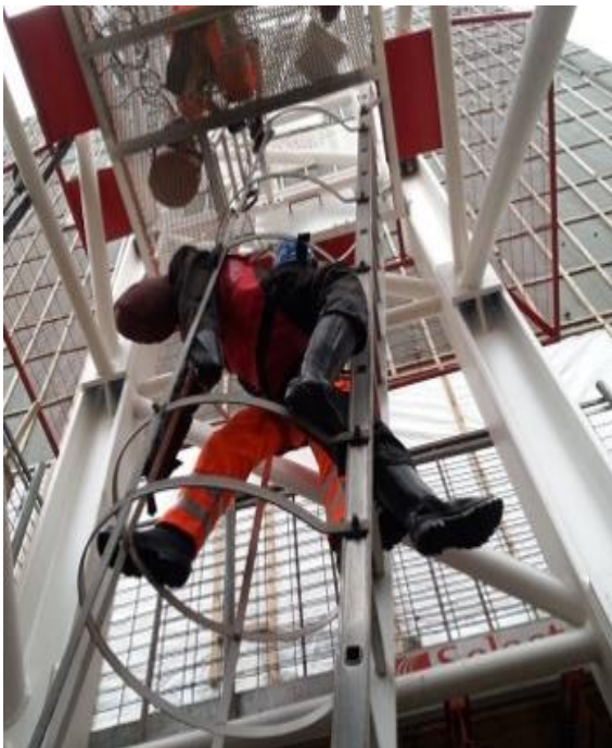
Figure 23: Rescue from within the mast sections
