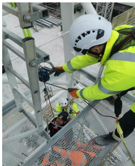
Figure 23: Rescue from within the mast sections
