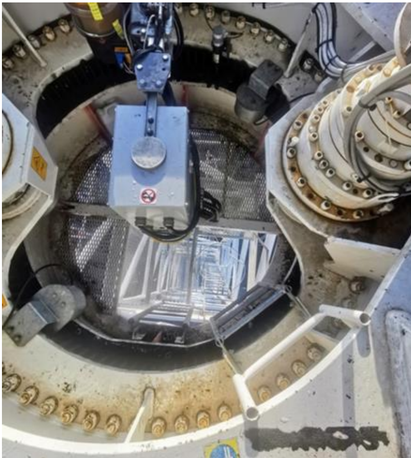
Figure 11: Restricted access through the opening at slew ring section
