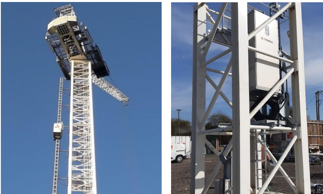
Figures 2: Example of a Passenger Lift
